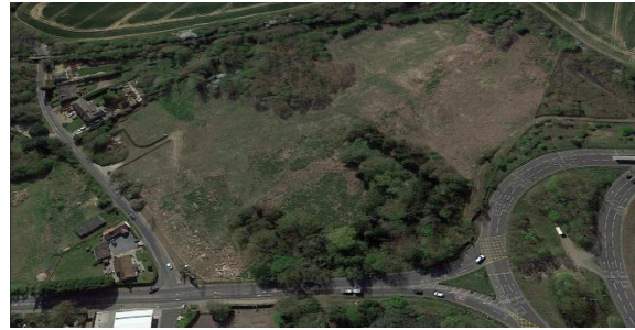
Site after tree cutting
