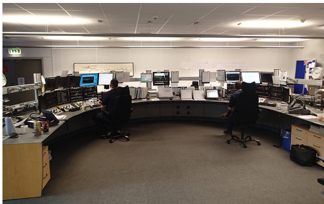
Operating floor at Cambrian line signalling control centre.
