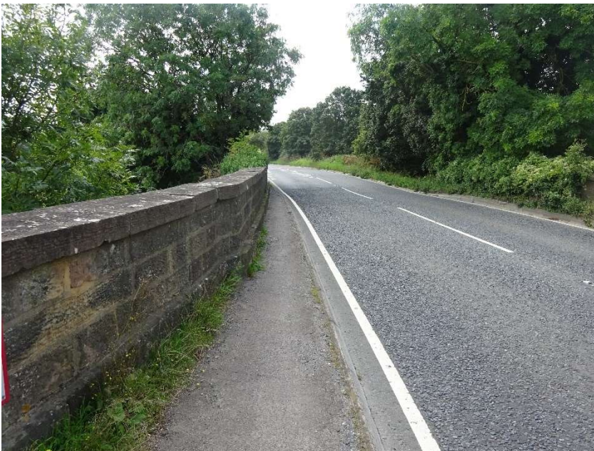
Plate 1: Existing Pedestrian Provision on A4135 Bridge over Railway Line
