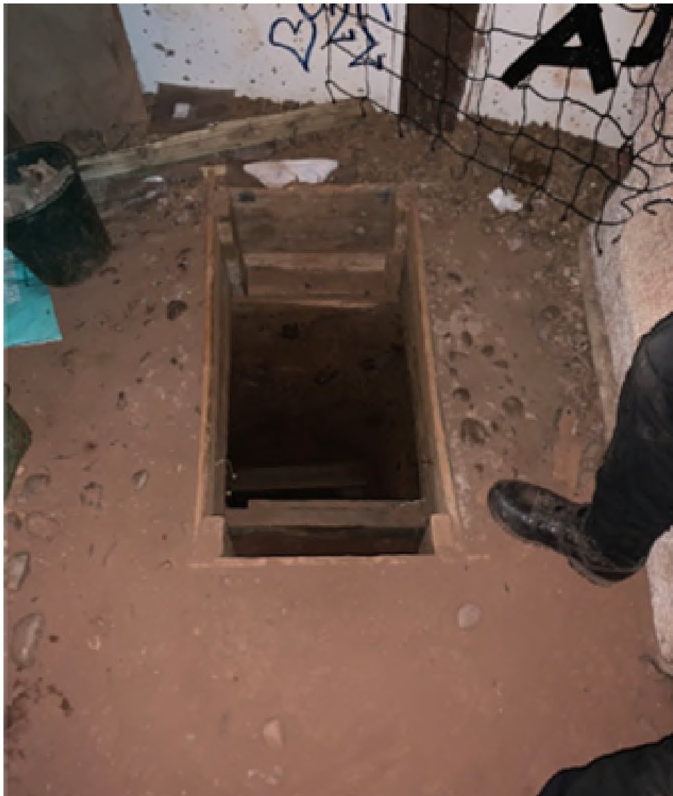
Main Tunnel head
