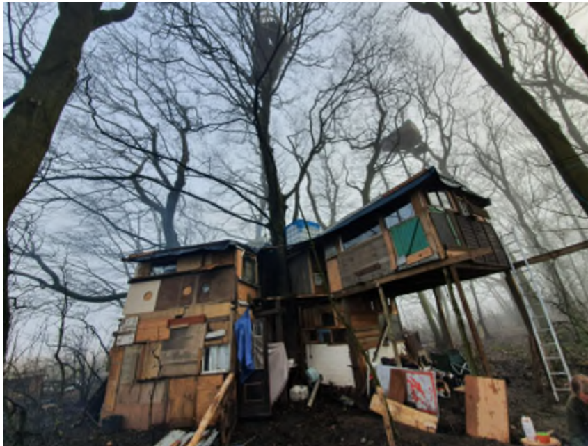
Photograph of NE structure in December 2021
