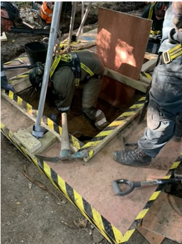
Tunnel removal team works on drop shaft
