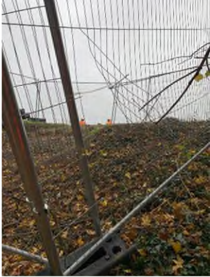
Damage to Heras fence
