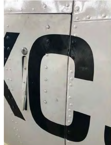
Protruding state of the lower cabin door handle observed during testing (image courtesy of 2Excel)
