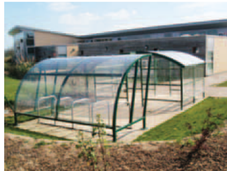
Secure and covered cycle parking within the grounds of a school
