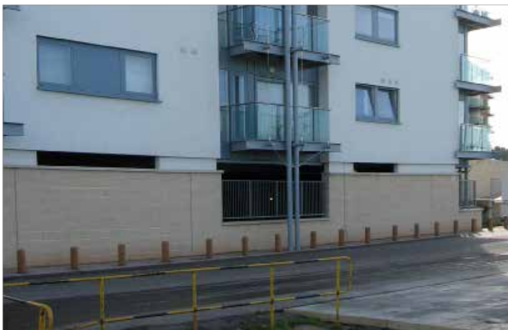
Poorly designed under-croft parking creates dead fronts and divorces the building from activities on the street
