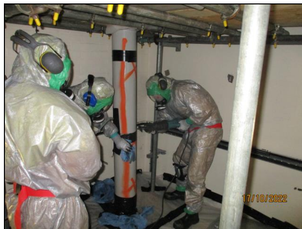
Photograph 8: De-plant of pipework
