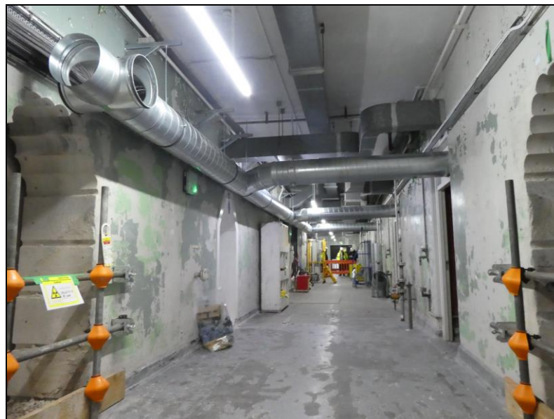
Photograph 11: Pond Filtration Plant
