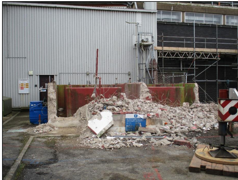
Photograph 16: Removed acid and caustic tanks
