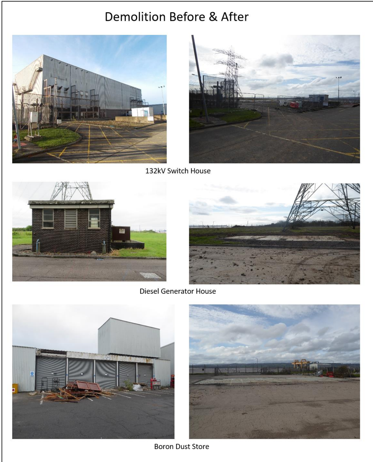
Figure 1: Images showing demolition progress
