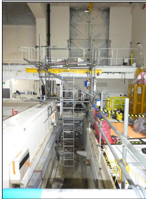
Photograph 9: Access arrangements to trench
