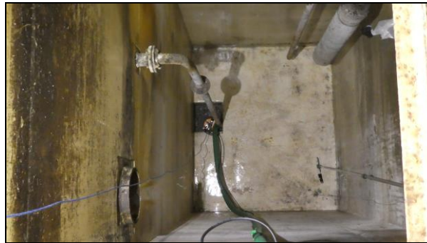
Photograph 7: Wet sump after decontamination
