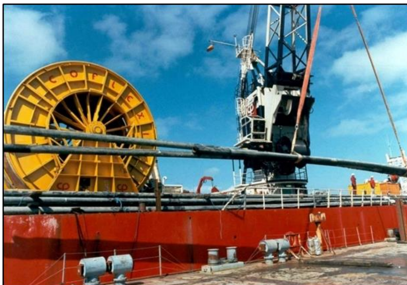
Figure 9: Pipeline Cut into Sections for Recovery
