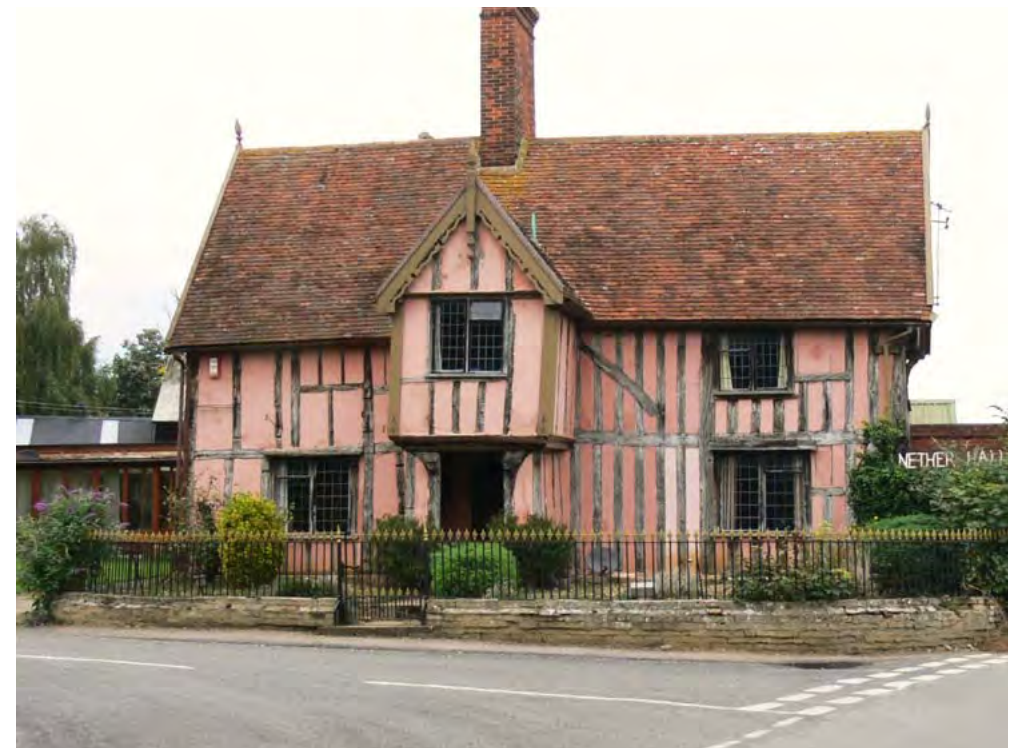
The Grade II listed 14th century Nether Hall in Cavendish is typical of many of the timber-framed medieval buildings that are a key characteristic of the area.
