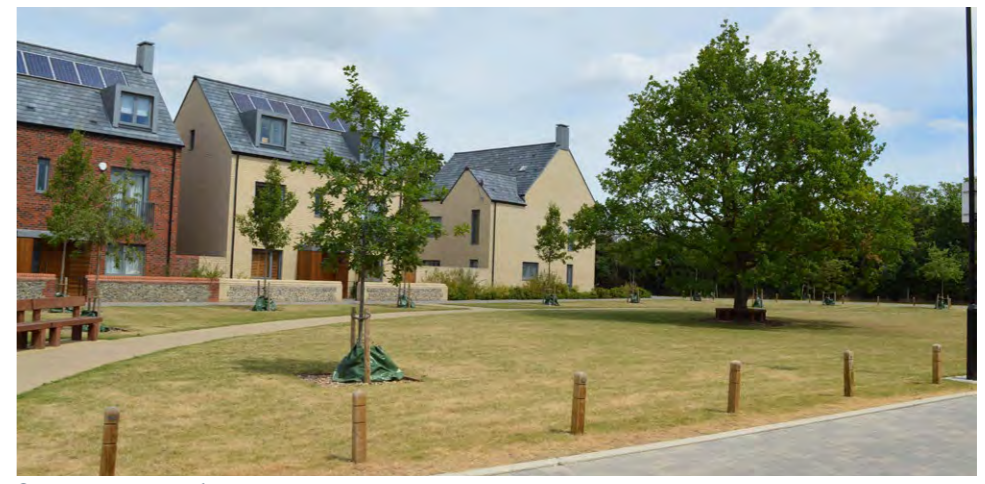
SINGLE-ASPECT DRIVE/LANE IN BLOCK PAVING OVERLOOKING OPEN SPACE, PROTECTED BY BOLLARDS
