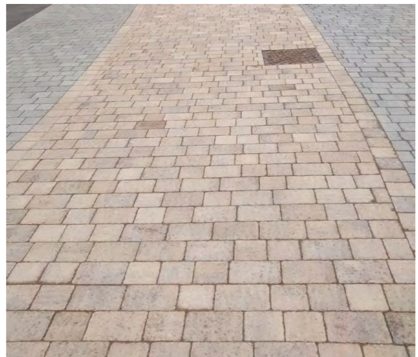
PERMEABLE PAVING TO LOOP ROAD
