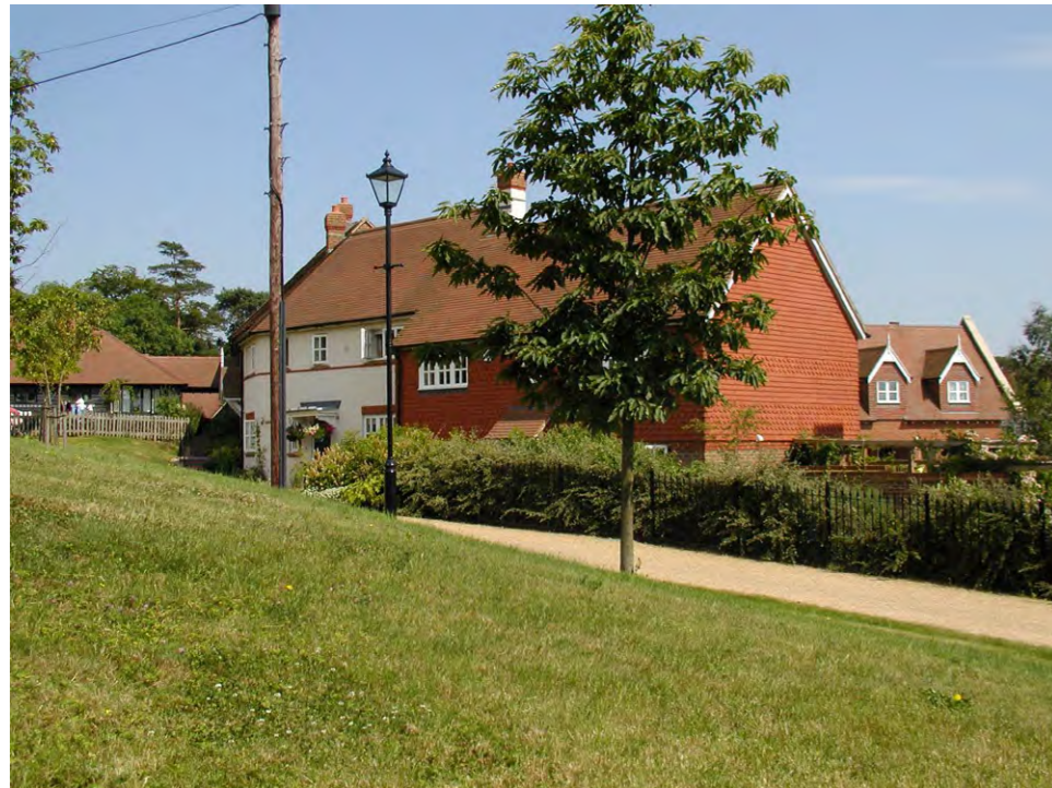
METAL RAILINGS FRAMING PRIVATE DRIVES AND OPEN SPACE
