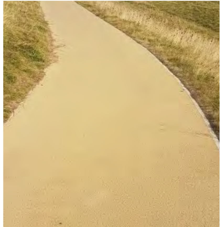
COLOURED TARMAC FOOT AND CYCLE PATH
