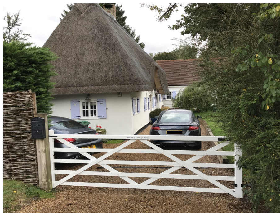
Figure 19: Hollow Elm Cottage (source: RPS photograph)
