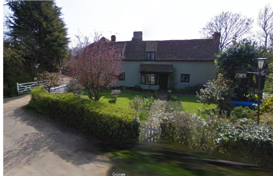
Figure 21 Cheerups Cottage (source: RPS photograph)
