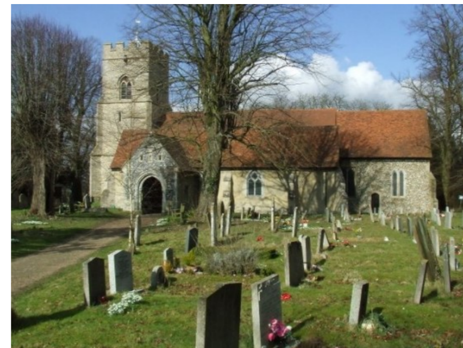
Figure 5: Grade I listed Church of the Holy Trinity (NHLE:1168843). (source: RPS photograph)
