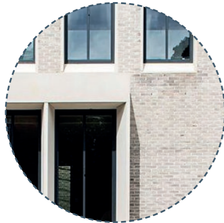
RENDER AND BRICKWORK
