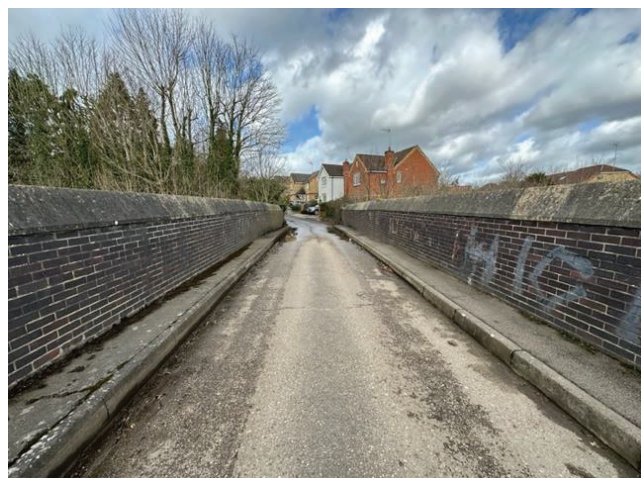
Stoney Common Road, shared surface over railway line
