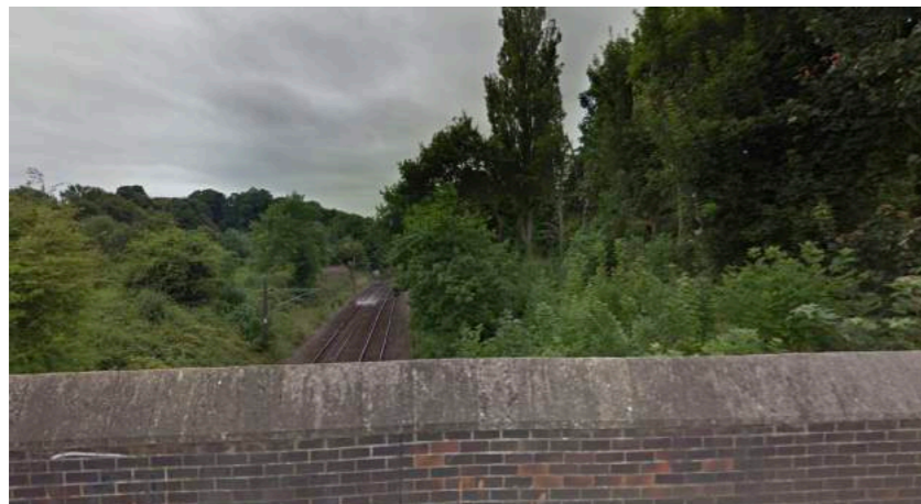
View of adjacent railway line
