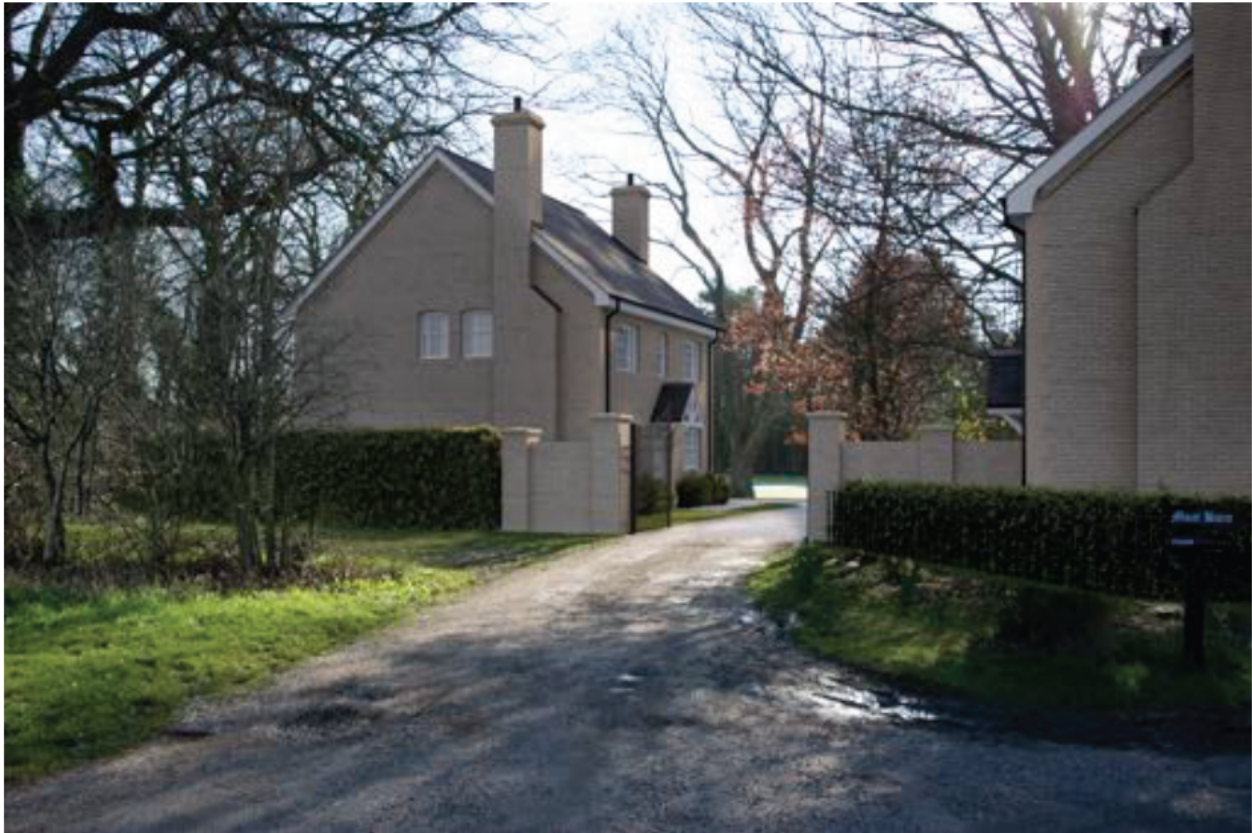
Gatehouse development (Units 1 & 2)
