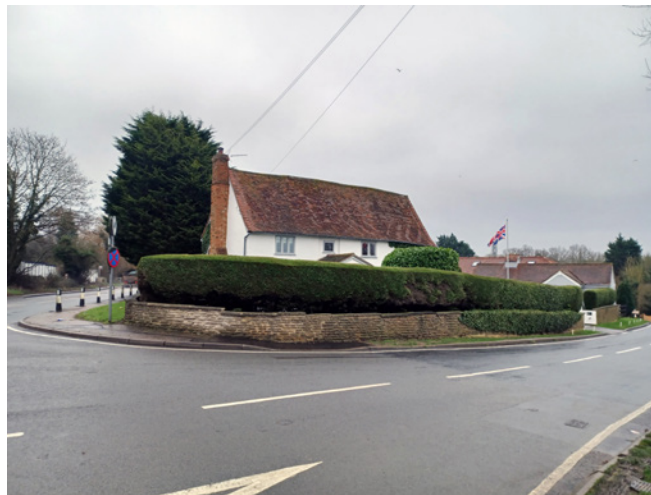
The north and west elevations of The Old Elm
