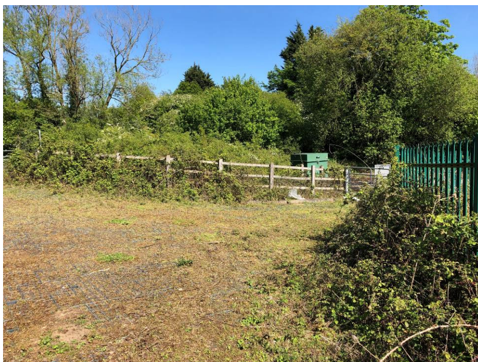
Plate 2.4 Foul water pumping station adjacent to eastern side of site, looking south east
