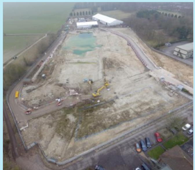
Figure 23: Harwell LETP footprint at March 2021
