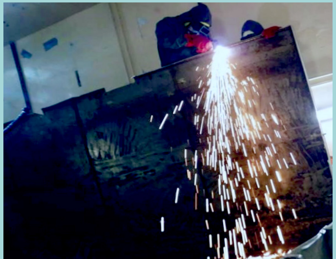
Figure 6: Operatives size reducing a tank from the AETP
