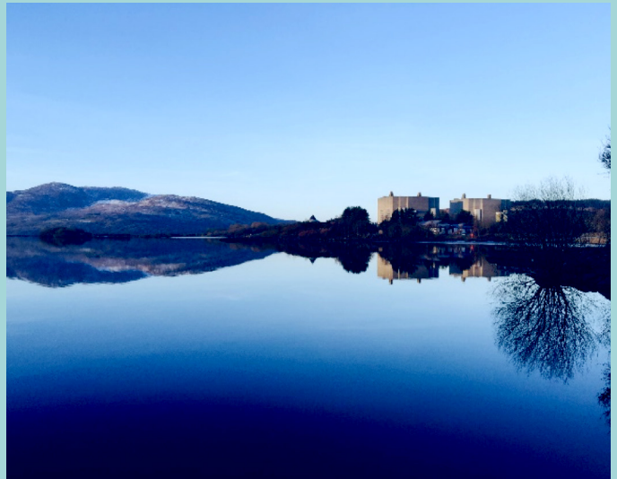
Figure 5: Trawsfynydd reactor buildings overlooking the lake
