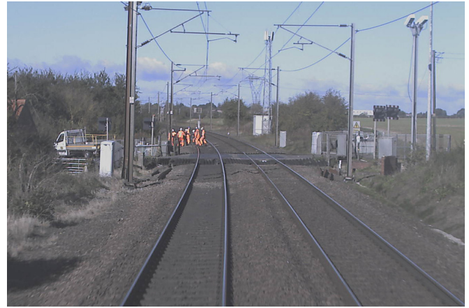
The work group clearing the line at Egmonton, less than two seconds before a train reached the place where they had been working.
