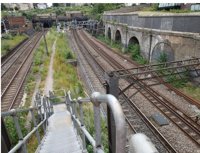
The view of the two sets of lines at South Hampstead from the access steps.
