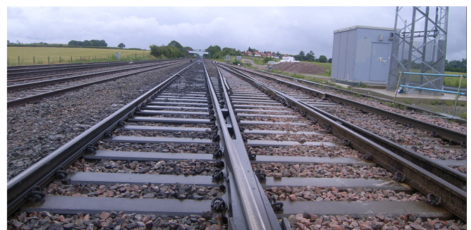
The site of the fatal accident at Ruscombe Junction.
