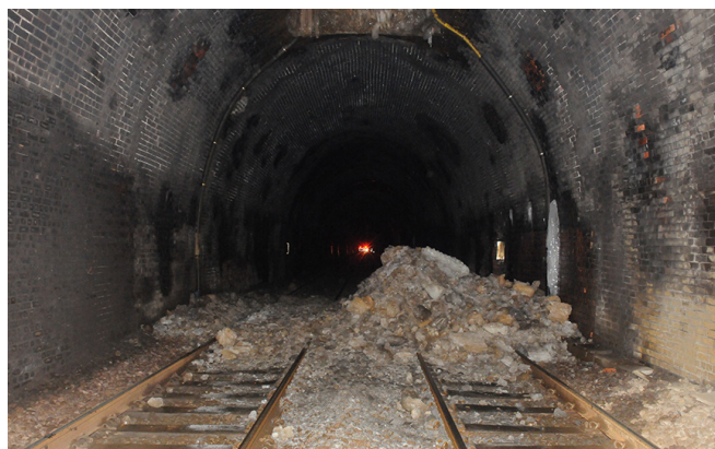
Ice found below a ventilation shaft after the derailment at Summit tunnel (courtesy of British Transport Police).
