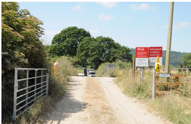
A user worked level crossing in Wales. Gates being left open is a regular problem at some crossings.
