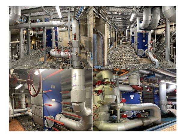
Pictures showing New Plate Heat Exchangers installation
