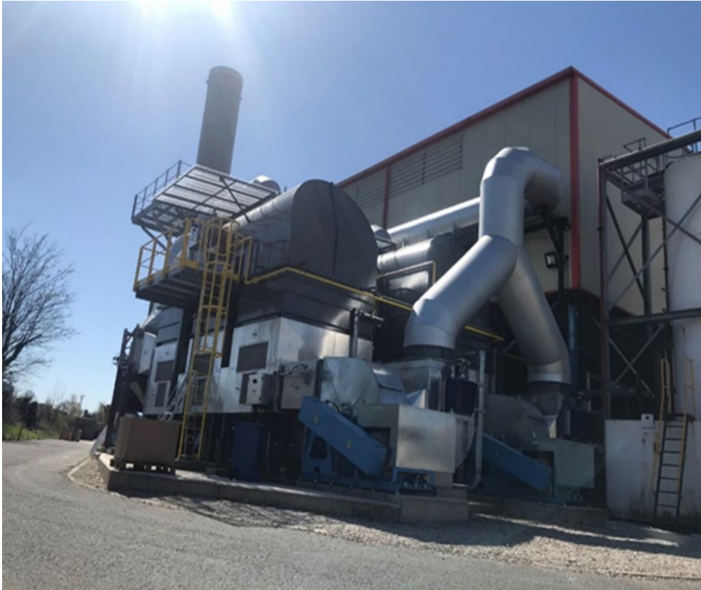
Picture of RTO where waste heat recovery is possible
