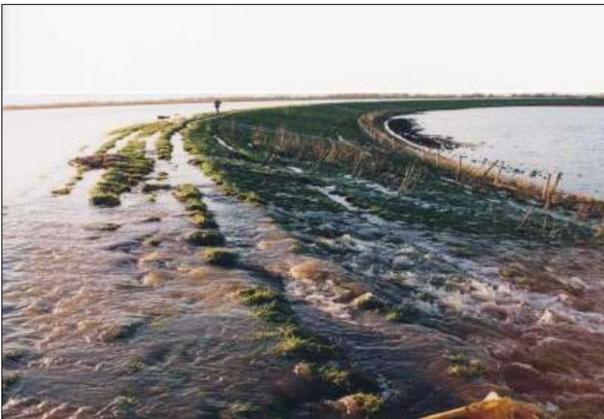
Figure 25 - Photo showing grass erosion: overflow at a depression in the crest initiating erosion at weak points in landward slope grass cover
