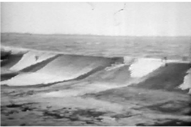
Figure 36 - Photo of waves overtopping across landward face of a coastal levee
