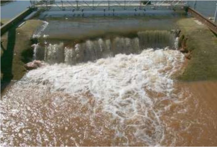
Figure 7 - Image of headcut advance through the embankment crest
