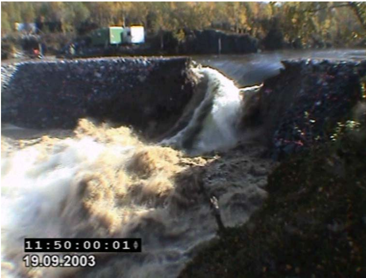
Figure 14 - Image of breach expansion during reservoir drawdown
