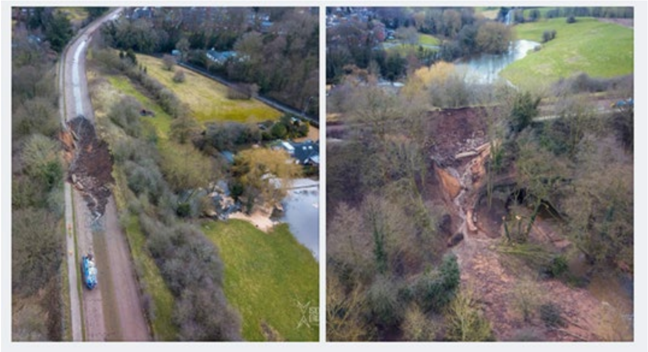
Figure 40 - Image of Middlewich Canal breach, March 2018
