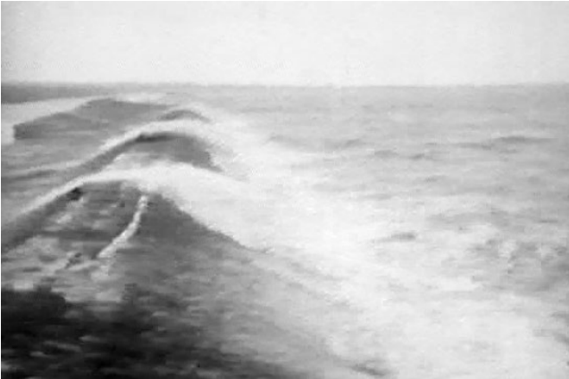
Figure 35 - Photo of waves impacting exposed face of a coastal levee
