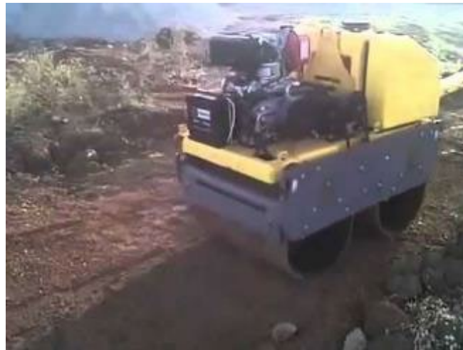
Figure 6.34: Tools for compaction in areas with limited access
