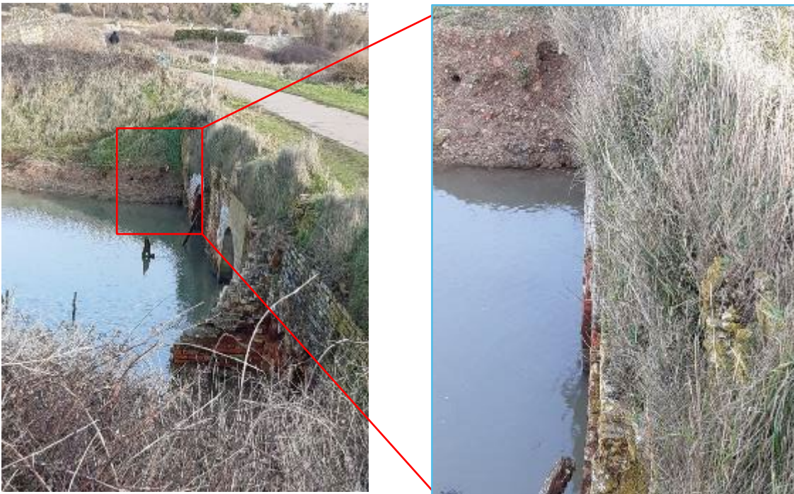
Figure 6.43: Animal burrows at transition with headwall, Tide Mills, Sussex, 2021
