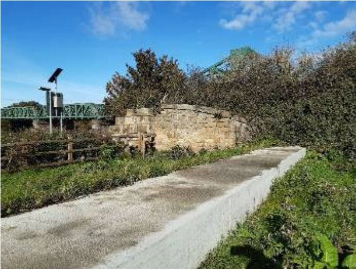
Figure 6.13: Type 1 transition – different assets with different geometries can lead to turbulence, south of Scunthorpe (Tidal River Trent), 2020
