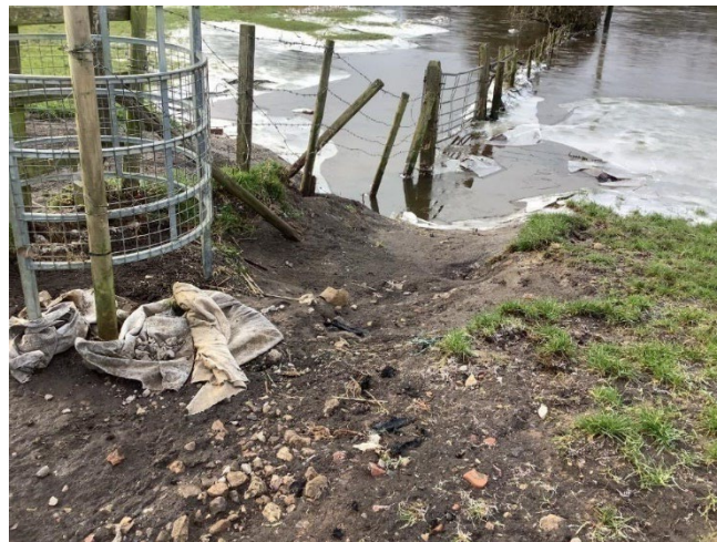
Figure 6.42: Preferential path alongside timber post and rail fence and gate, Kirkby Wharfe, 2021
