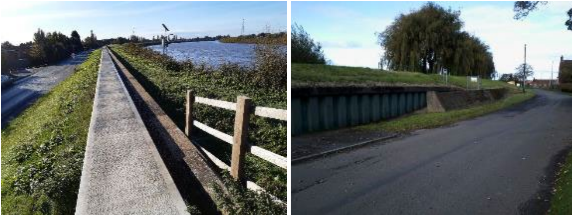
Figure 3.3: Type 2 transition examples (at south of Scunthorpe and East Butterwick (Tidal River Trent), 2020)
