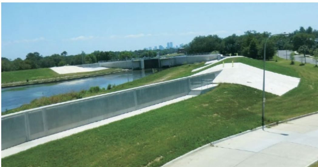
Figure 6.20: ILH Figure 3.149 Gradual transition between wide levee and narrow floodwall, New Orleans, Louisiana, USA (courtesy USACE)
