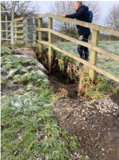
Figure 6.42: Preferential path alongside timber post and rail fence and gate, Kirkby Wharfe, 2021
