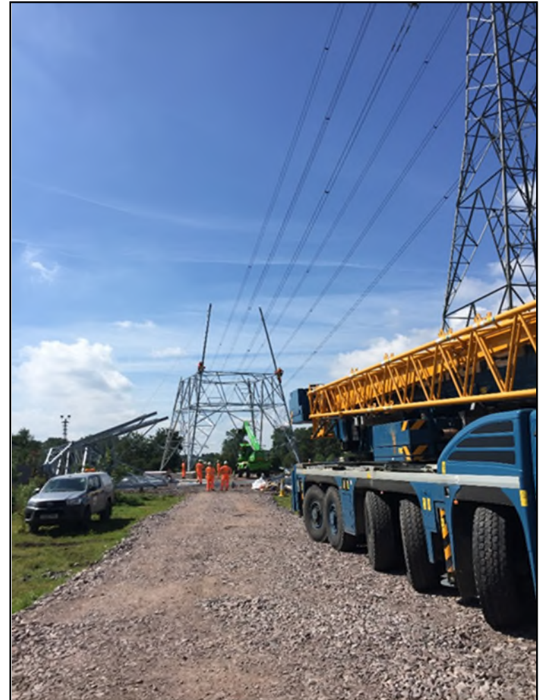
HS2 Phase One, works between Birmingham Interchange and Hints (Tamworth)
