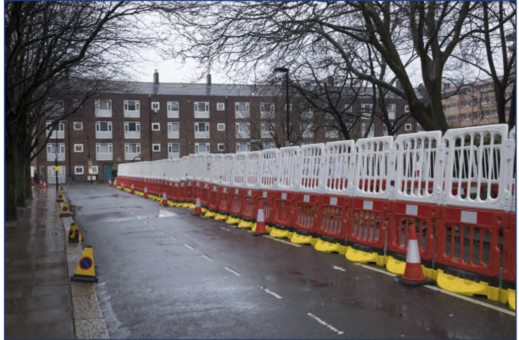
HS2 Phase One, works at Euston
