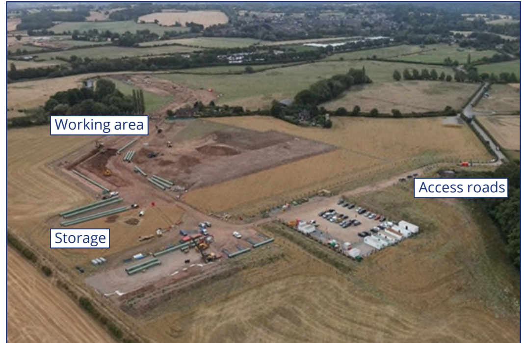
HS2 Phase 2a, National Grid works near Kings Bromley
