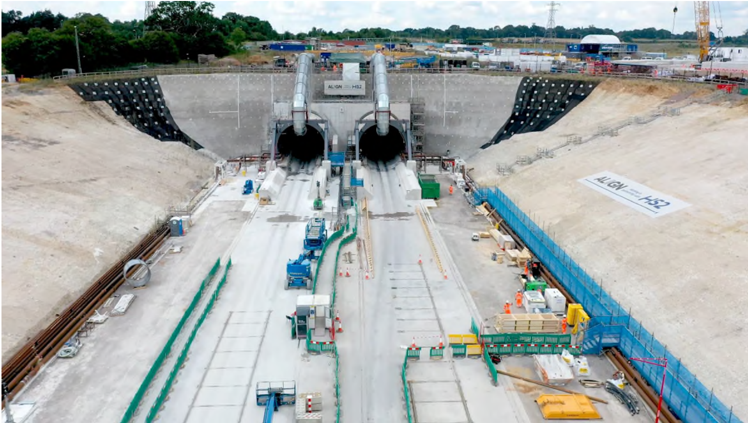
Bored Tunnel - Chiltern Tunnel South Portal
