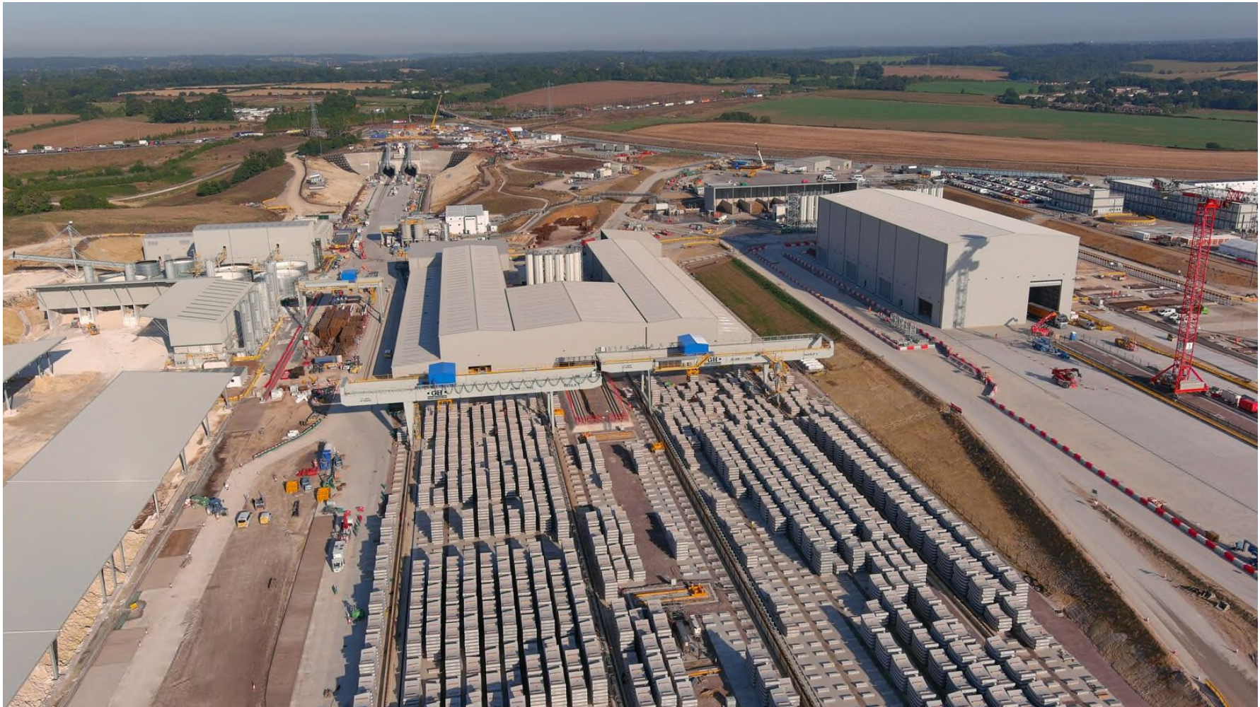
South Portal Site (Chiltern Tunnel), Phase One
