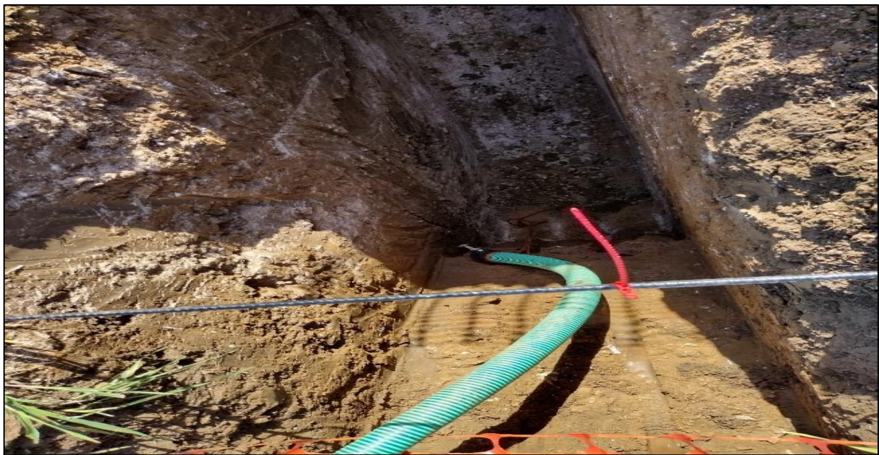
Photo 2 Pit SA101A : Example of Head deposit.
