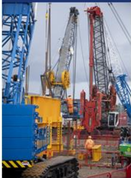
Phase One construction
