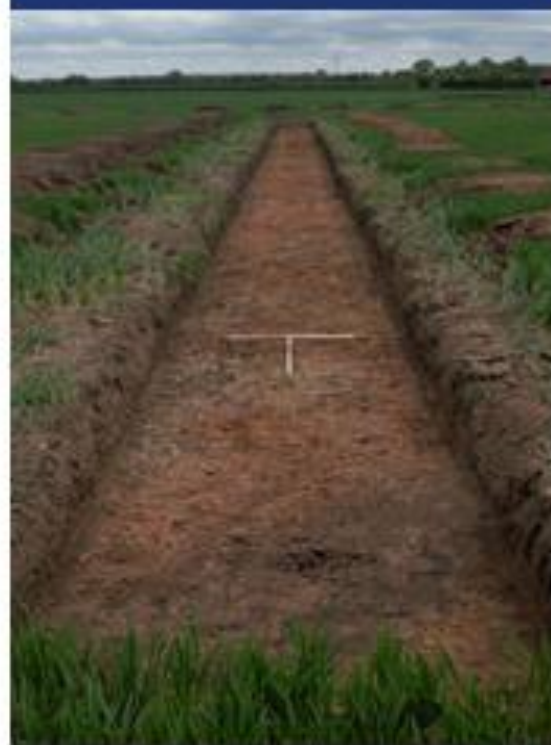
Phase 2a enabling works
