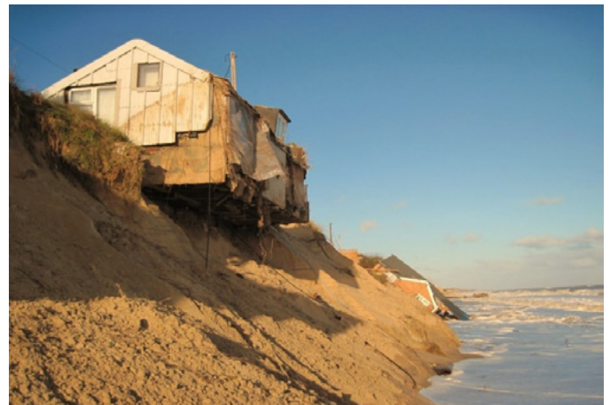
The impacts of coastal erosion in Hemsby, Norfolk. Seven houses were lost during a storm surge in 2013.
