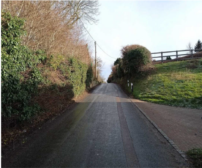
Photo 4: Section of narrow carriageway between Village Hall (just visible on left) and village showing blind crest
