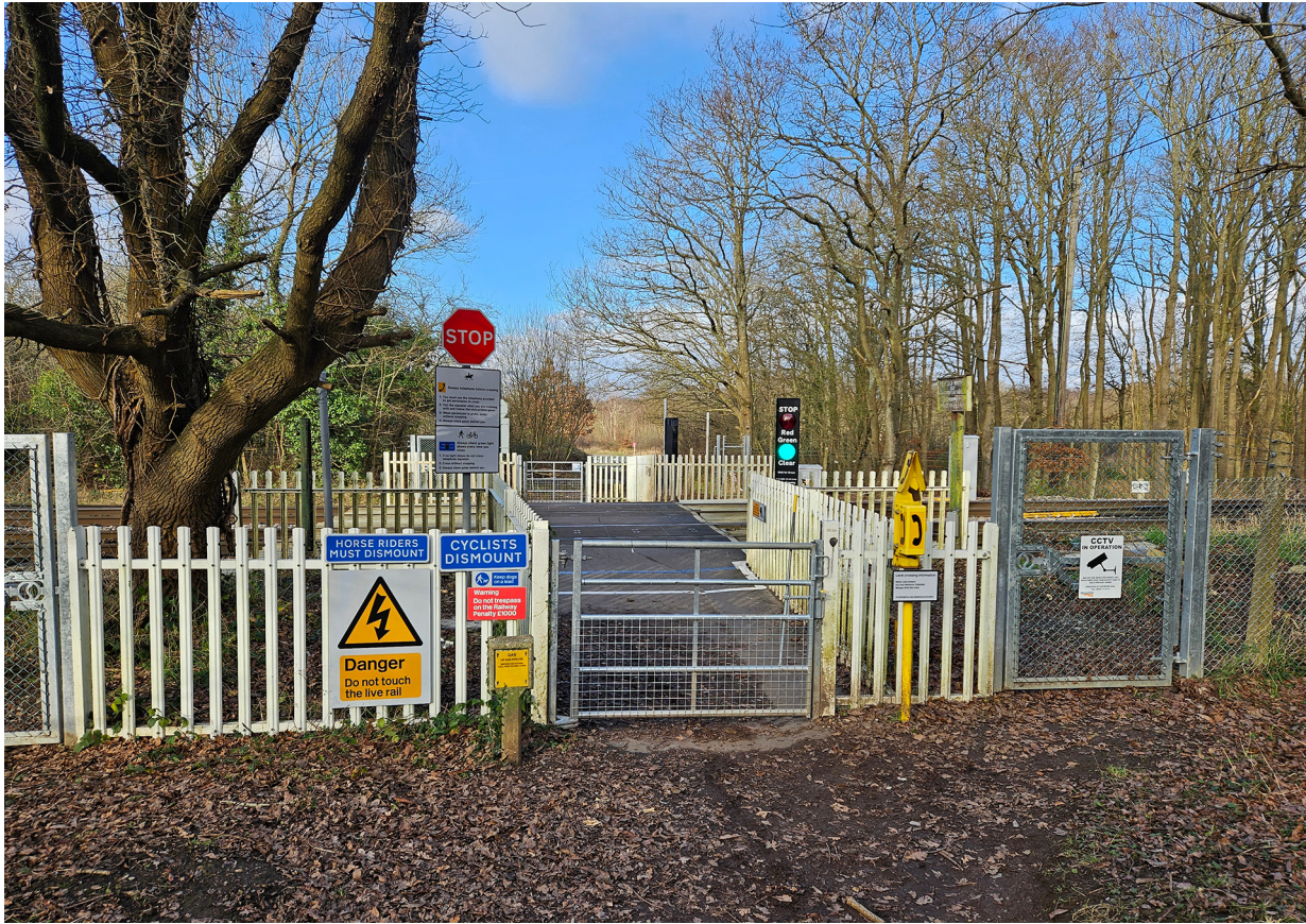
Figure 11: Lady Howard crossing, fitted with overlay MSLs (courtesy of Network Rail).
