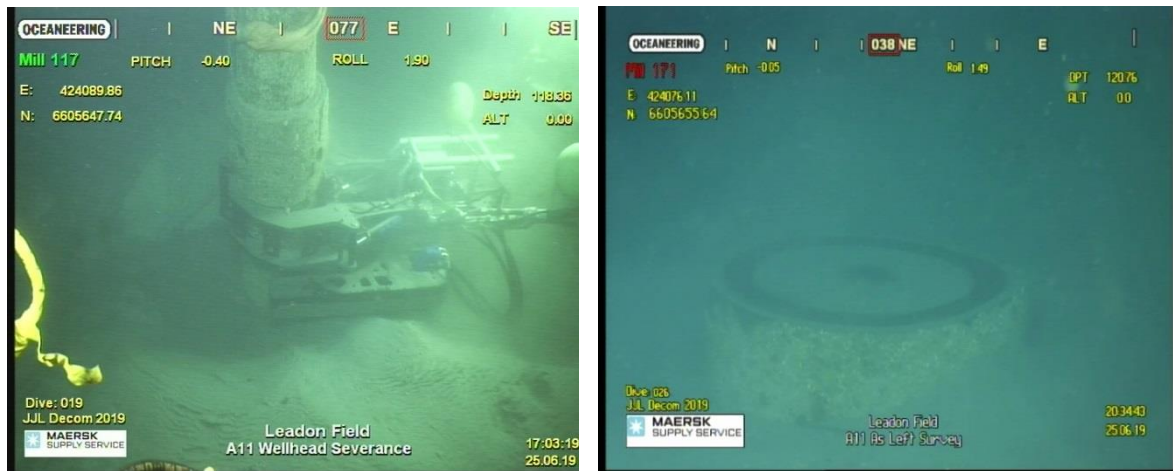
Figure 9: A11 Conductor Seabed Cutting
