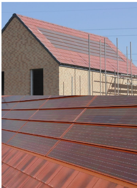
Integrated photovoltaic clay-type roof tile (source: Romag)
