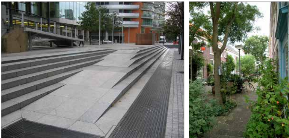
(right) Wheelchair and pushchair ramp incorporated with steps, Paddington Basin, London Image
