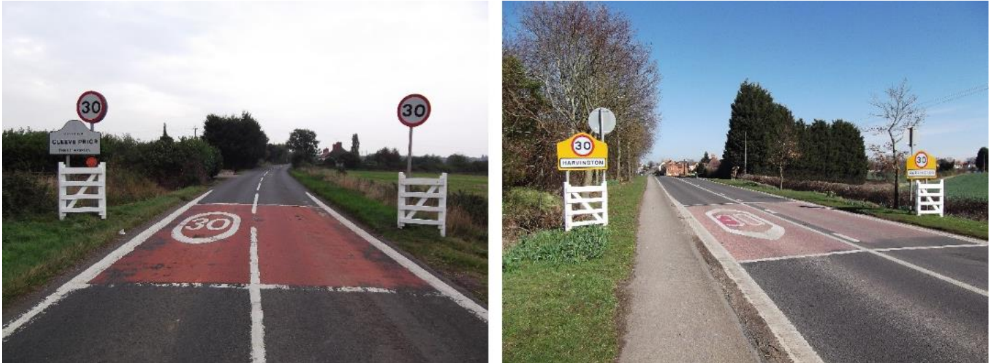
Figure 1: Examples of Gateway Features installed in Worcestershire (source: jacsuk.com)
