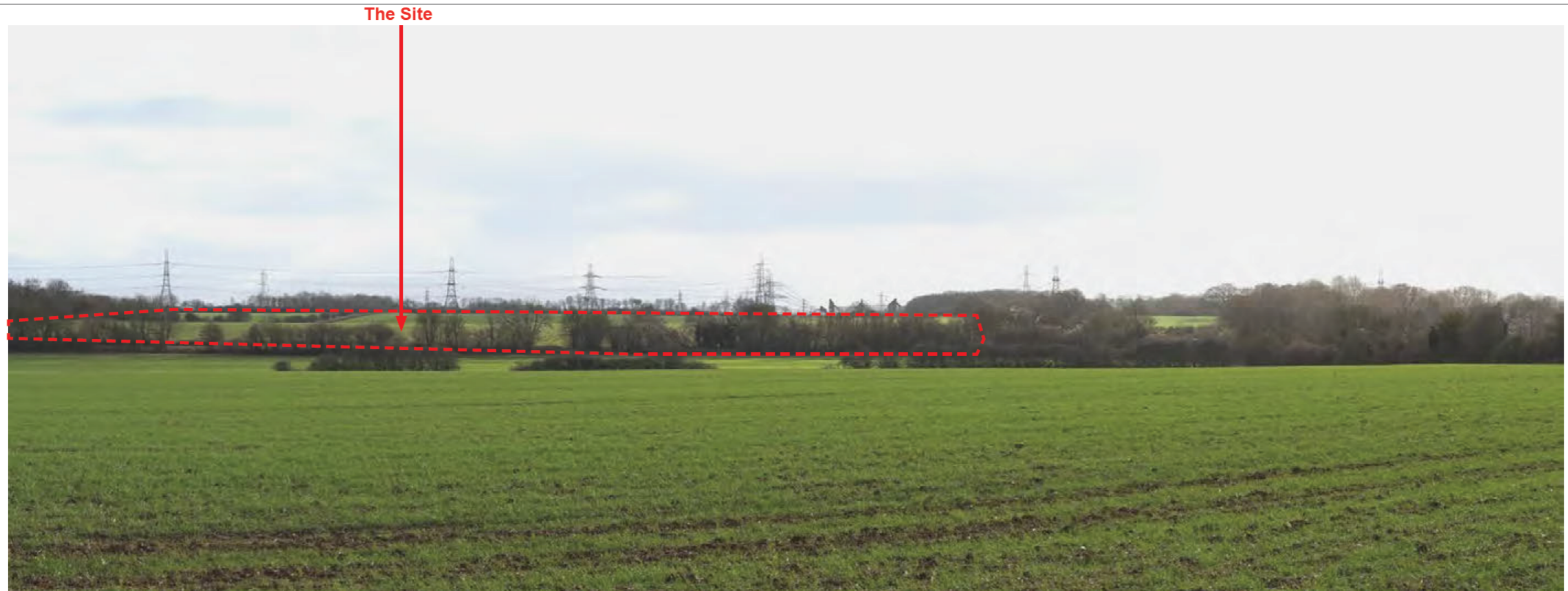
Figure 10.14: View from PRoW 5/29 which crosses slightly elevated ground south of the site (Panoramic View)
