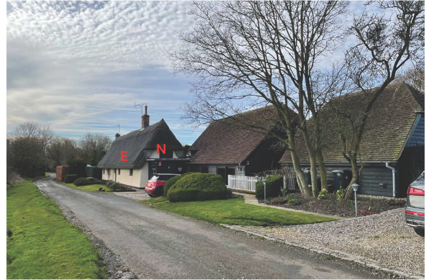
East and north elevations
