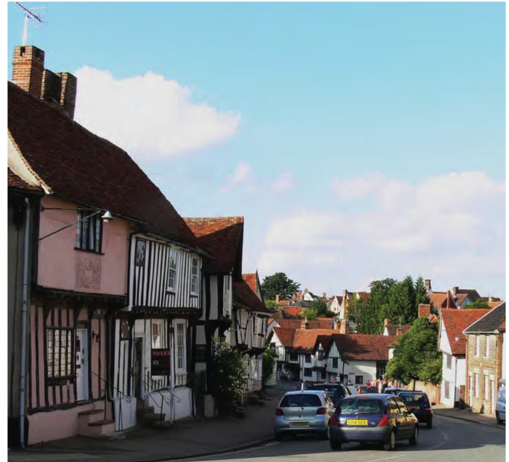
The well preserved medieval small town of Lavenham with its distinctive timber-framed, colour-washed buildings, that contribute to the rural sense of place, is a popular visitor destination.
