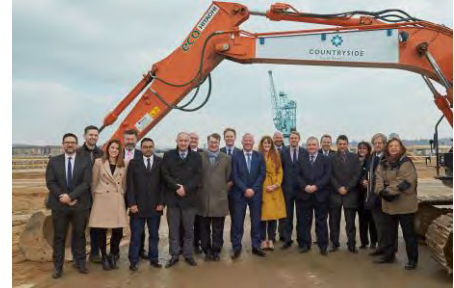
Rochester Riverside Ground breaking ceremony 22 March 2018
