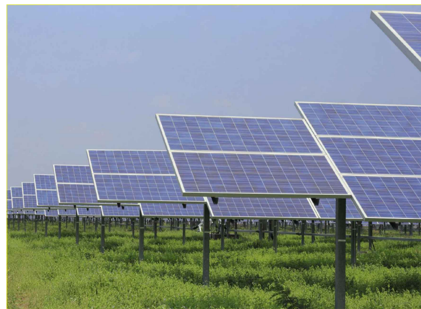
TYPICAL SOLAR PANEL ARRANGEMENT RAISED ABOVE GROUND
