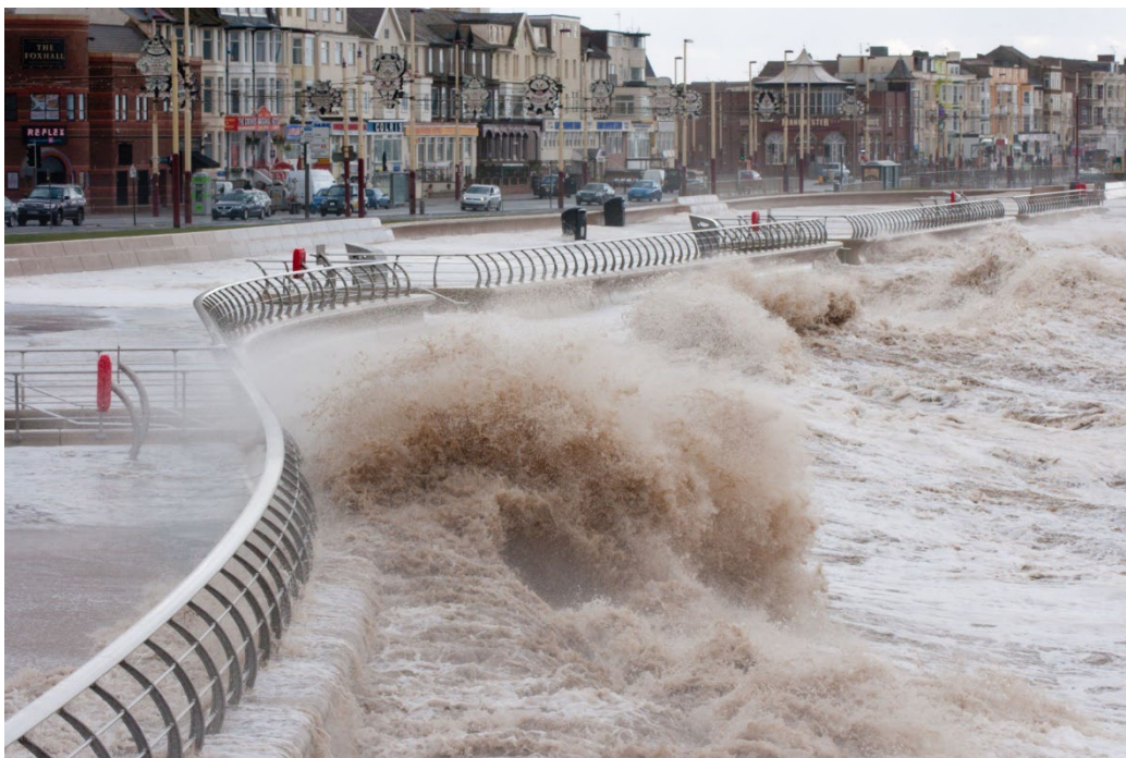
Photo 1: waves overtopping a sea wall
