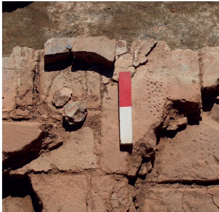
Detail view of hobnail impressions on tiles used in construction of Romano-British kiln 396216, view from north-east, 0.2 m scale
