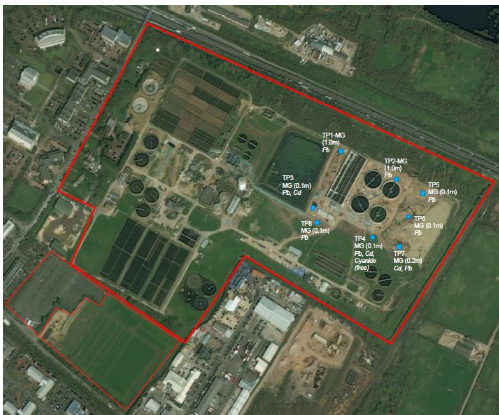
Above: Locations where soil contamination has been identified in previous site investigations
