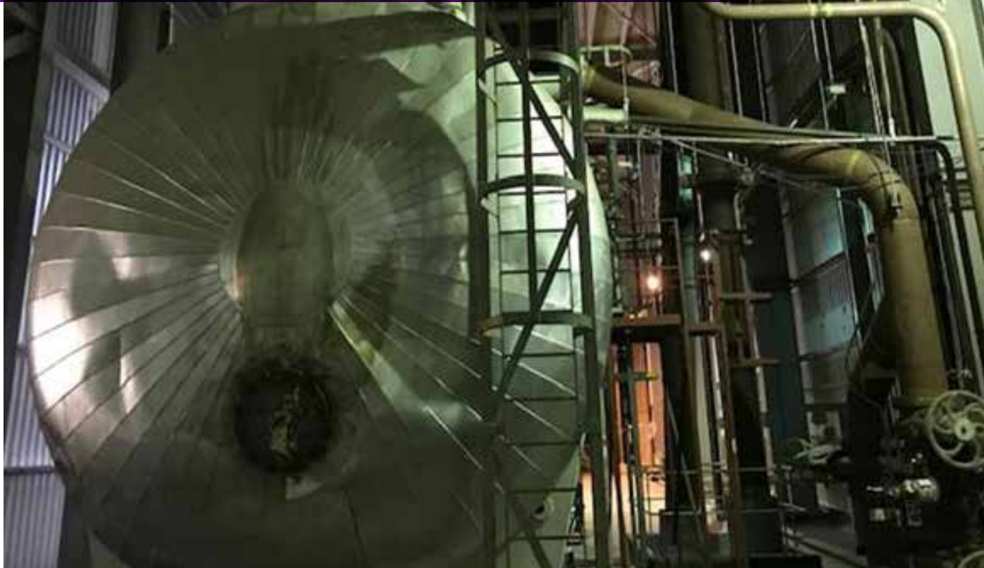
Asbestos removal at Wylfa
