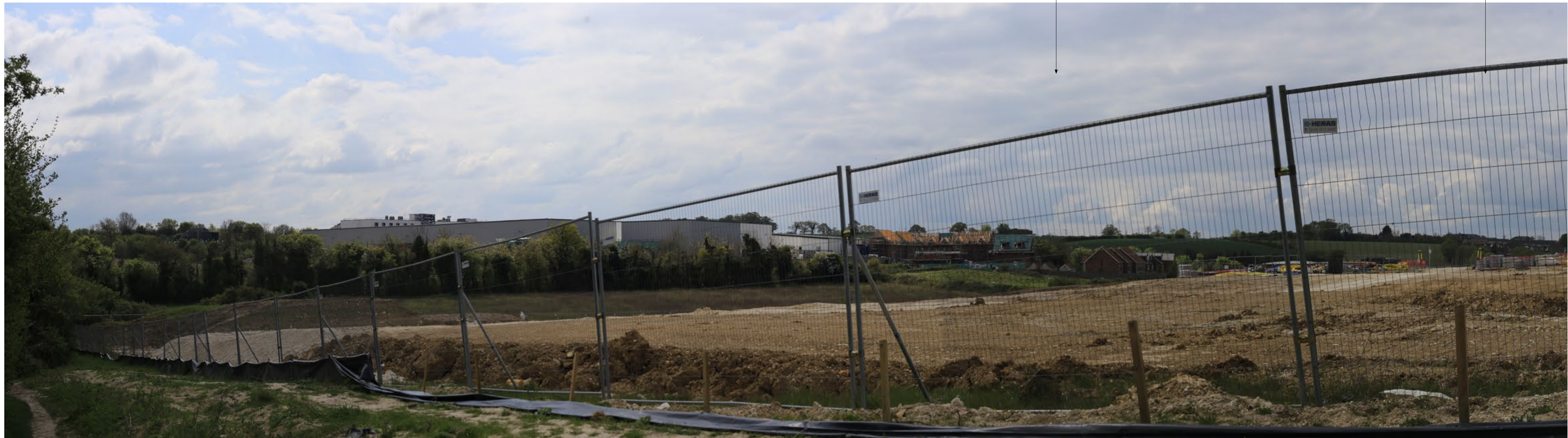
Viewpoint 13: Westerly view from public bridleway by the Bellway development
