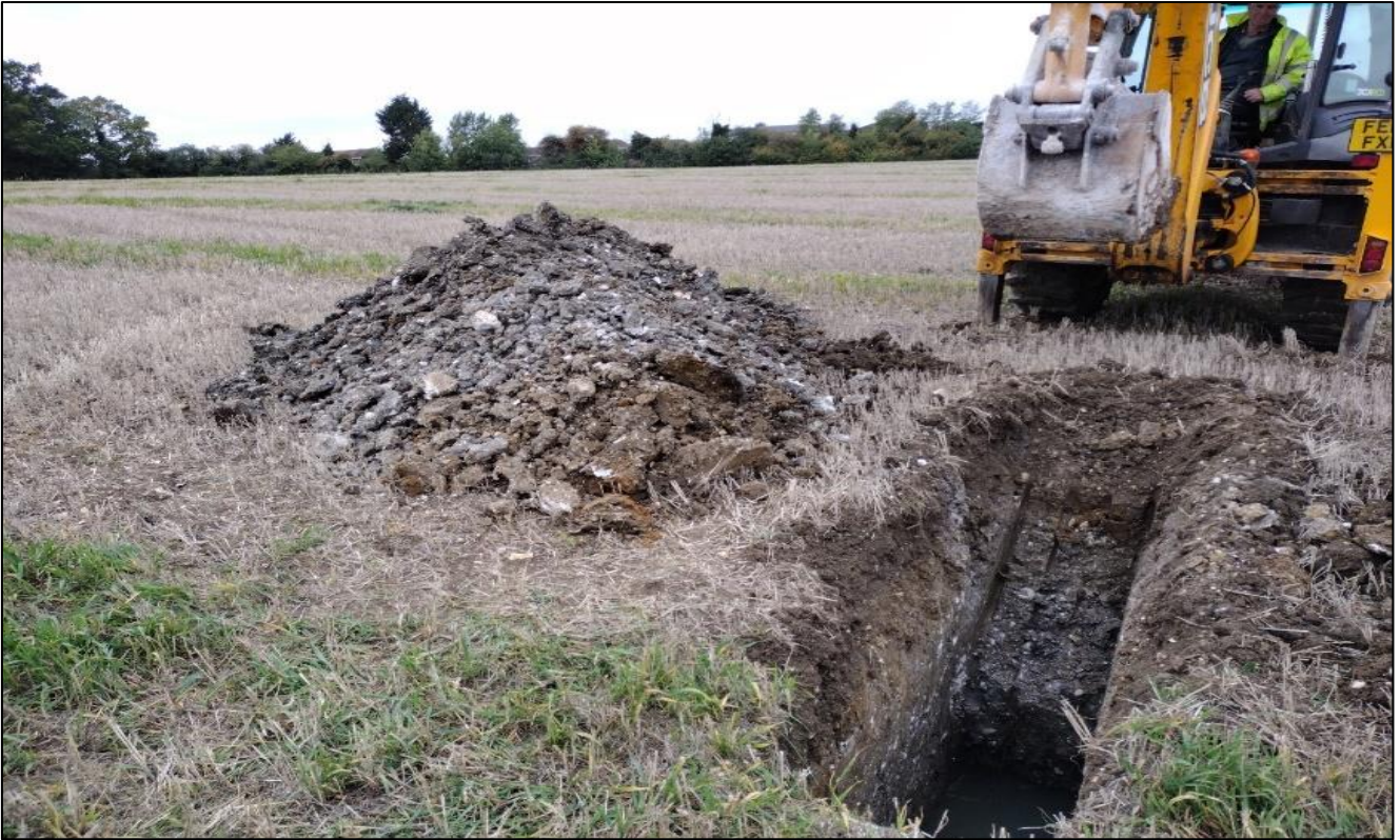
Photo 3 Pit SA107 : Example of Lowestoft Formation.
