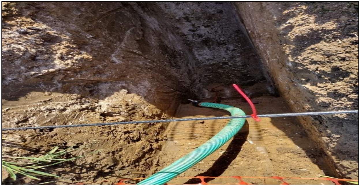
Photo 2 Pit SA101A : Example of Head deposit.
